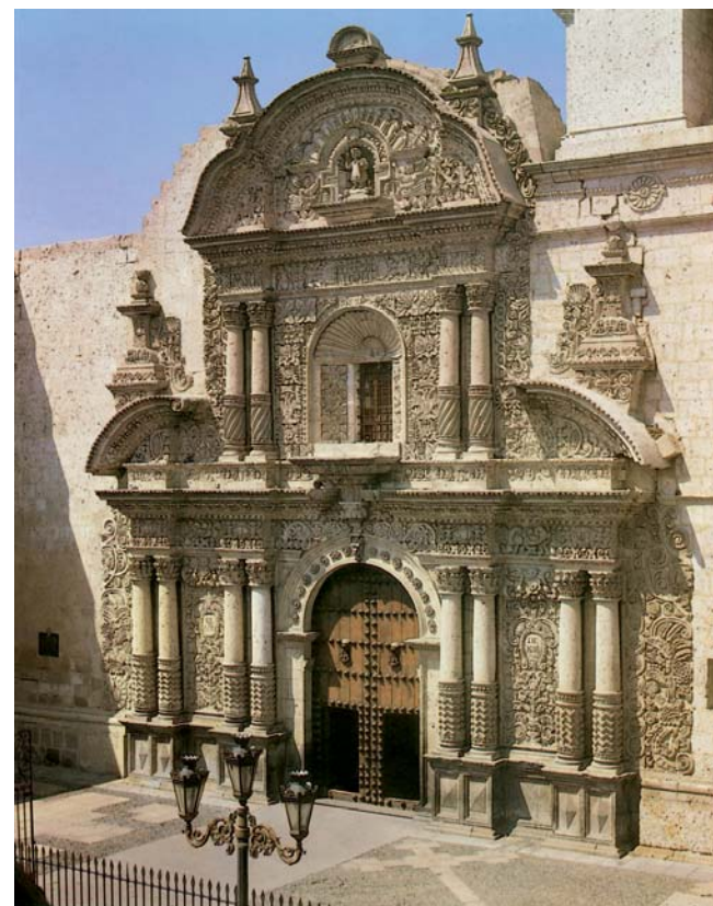
Facade, Church of the Company (Arequipa). Anonymous. IOPS. Sculpted sillar volcanic stone. Photo: Daniel Chamoni.
